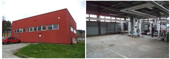
**VS92** is classic secondary exchange station supplying heating 90/70 PN 6 and hot water with central domestic hot water preparation in the heat exchange station (55°C) via 4-pipe pre-insulated pipeline into residential buildings.
