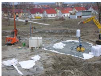
Figure 6: Drilling the boreholes
