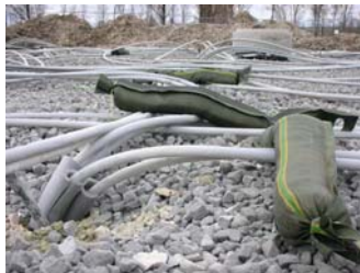
Figure 7: pipe installation in the boreholes and foam glass gravel insulation
