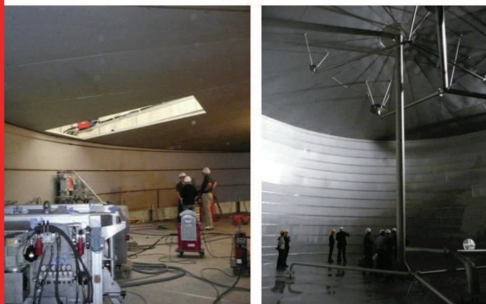
Realisation of multifunctional heat storage in Hamburg, 2010
