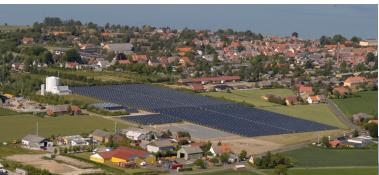
Solar district heating (SDH) plants are a large-scale solar thermal technology supplying renewable, zero-emission heat from large collector fields via district heating systems to residential and industrial areas.
