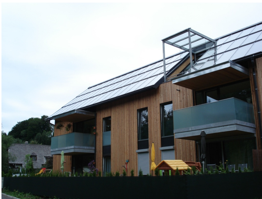
Fig. 2.2.7. Roof integration (Sonnenkraft), Austria [3].
