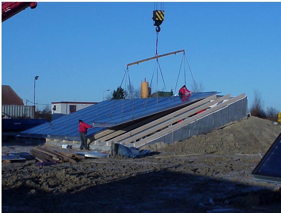
Fig. 2.2.6. Implementation of roof modules (Wagner), Marstal, Denmark [2].
