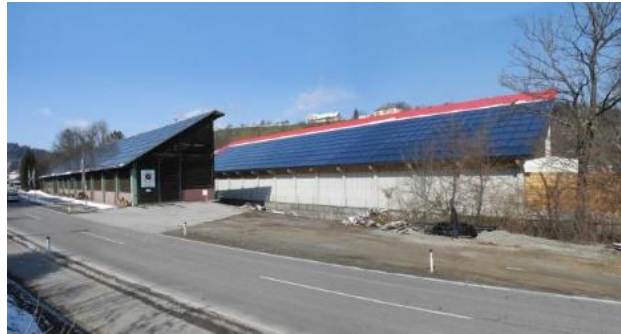
Fig. 1: Eibiswald district heating plant, a solar thermal frontrunner in Styria
