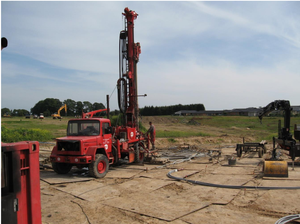
Fig. 11. Drilling of boreholes. Source: PlanEnergi
